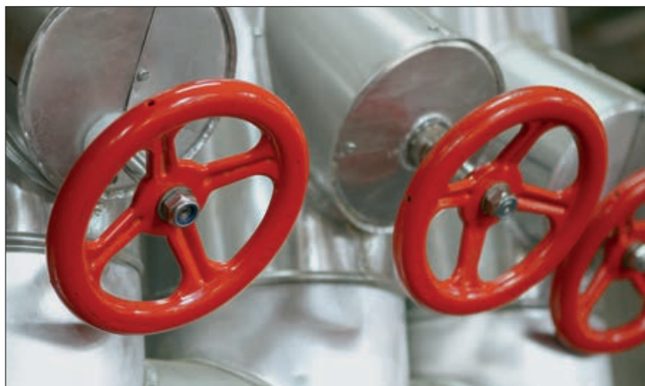
Fig. 38: Valve pressure test
